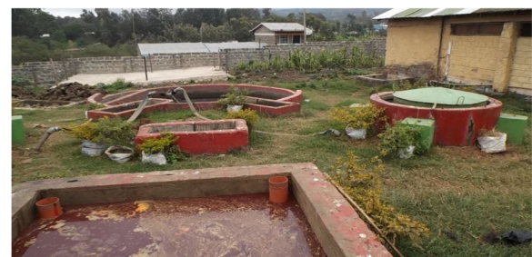
Fig. 6 Biogas generation system for managing liquid waste in a slaughterhouse in Kajiado County
