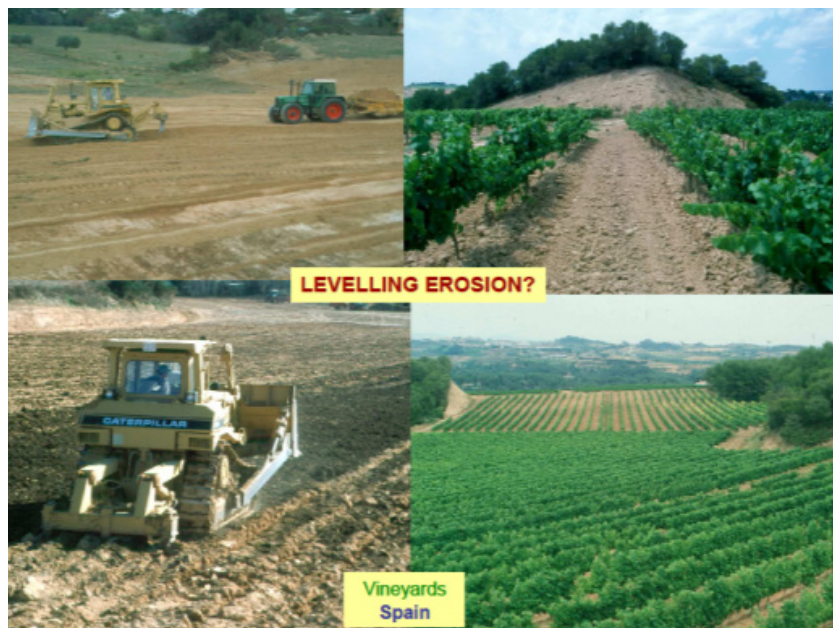
Figure 6. Soil displacement (tillage erosion? Leveling erosion?) caused by land leveling in vineyards (NE Spain) (Pla and Nacci 2011).
