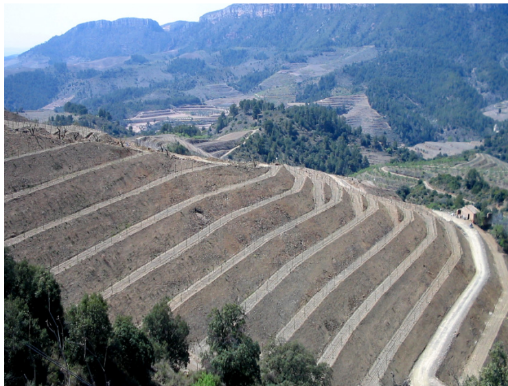
Figure 9. Bench terracing in vineyards (Priorat-NE Spain), promoted and subsidized with “European Community” funds for the control of surface erosion.
